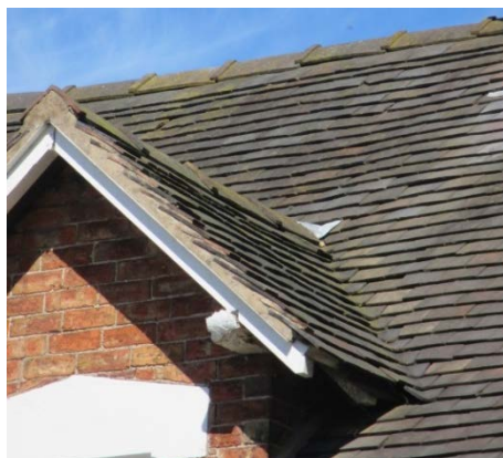
Staffordshire blue clay plain tiles typical of historic roofing
